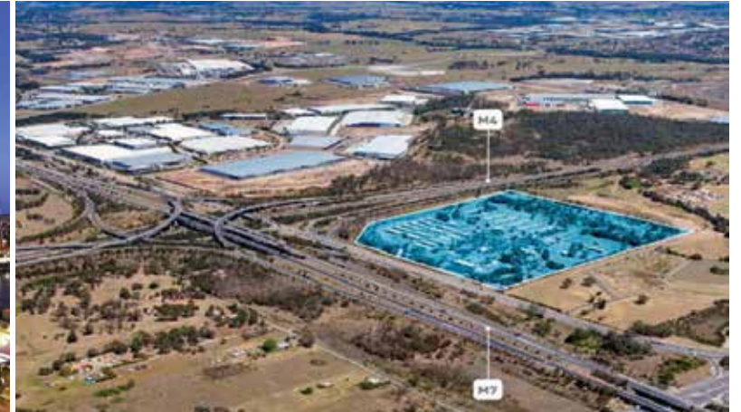
60 Wallgrove Road, Eastern Creek, NSW
